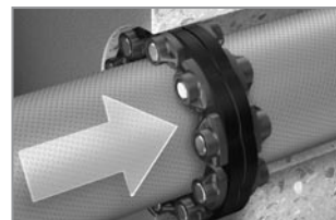
Push link chain into final position
